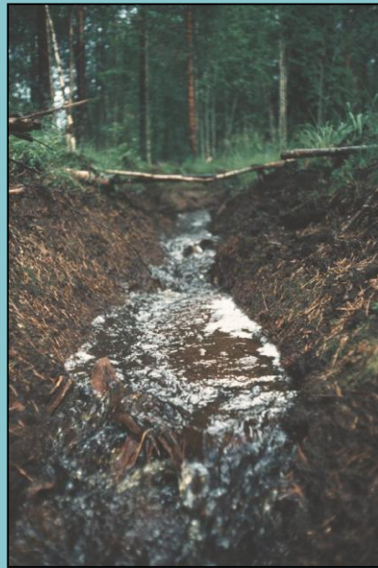
Ditch in peatland is more durable than ditch in sandy soil
