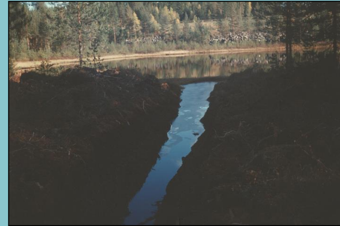
Ditch caused a permanent lowering of the water level in a lake
